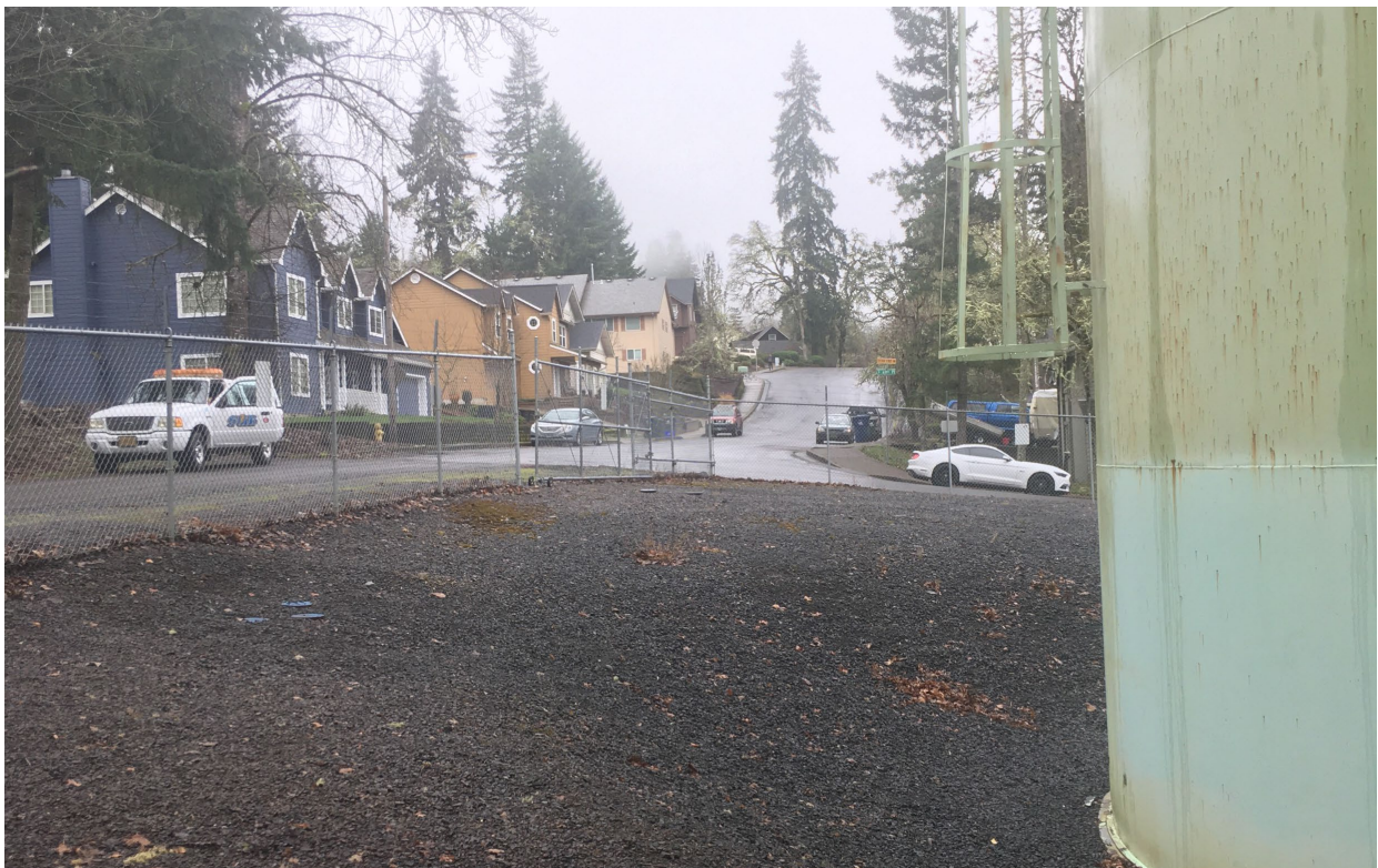
S 70 th Street Reservoir – Looking W
