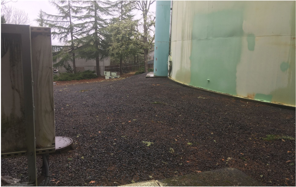
S 67 th Street Reservoir – Looking E
