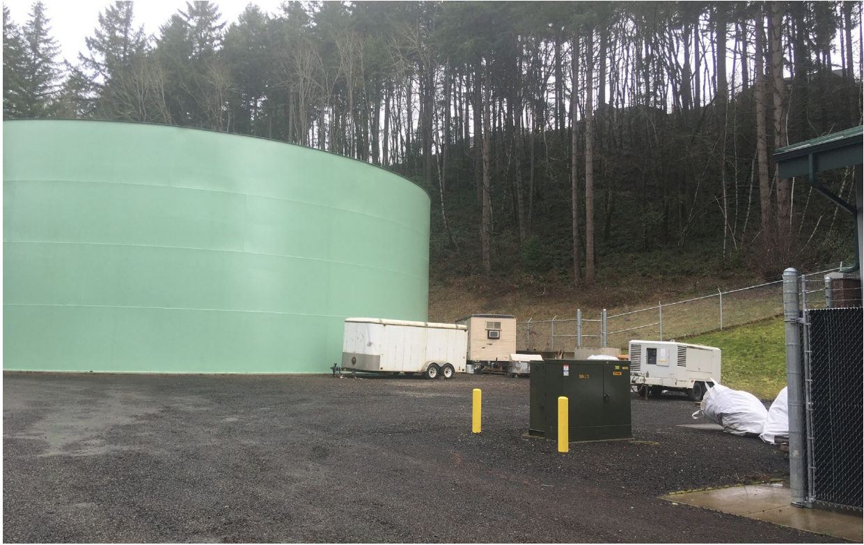
S 57 th Street Reservoir – Looking NE
