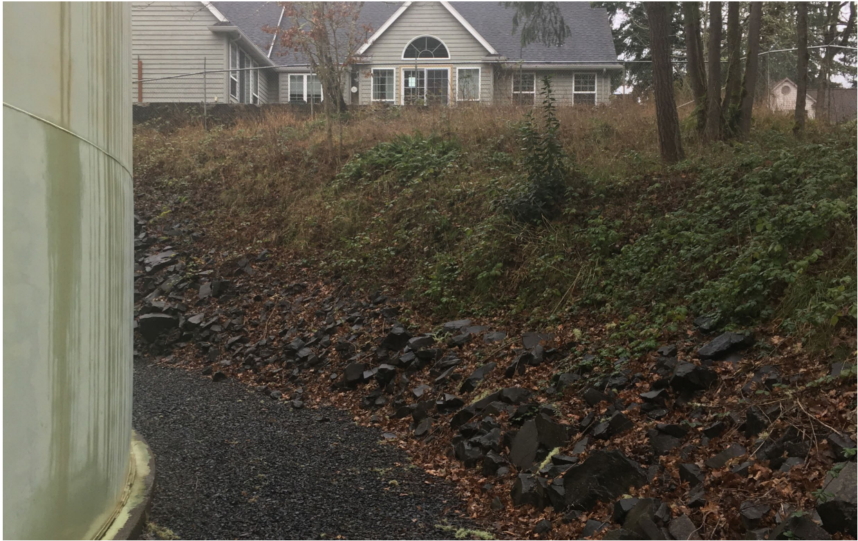
S 67 th Street Reservoir – Looking NE
