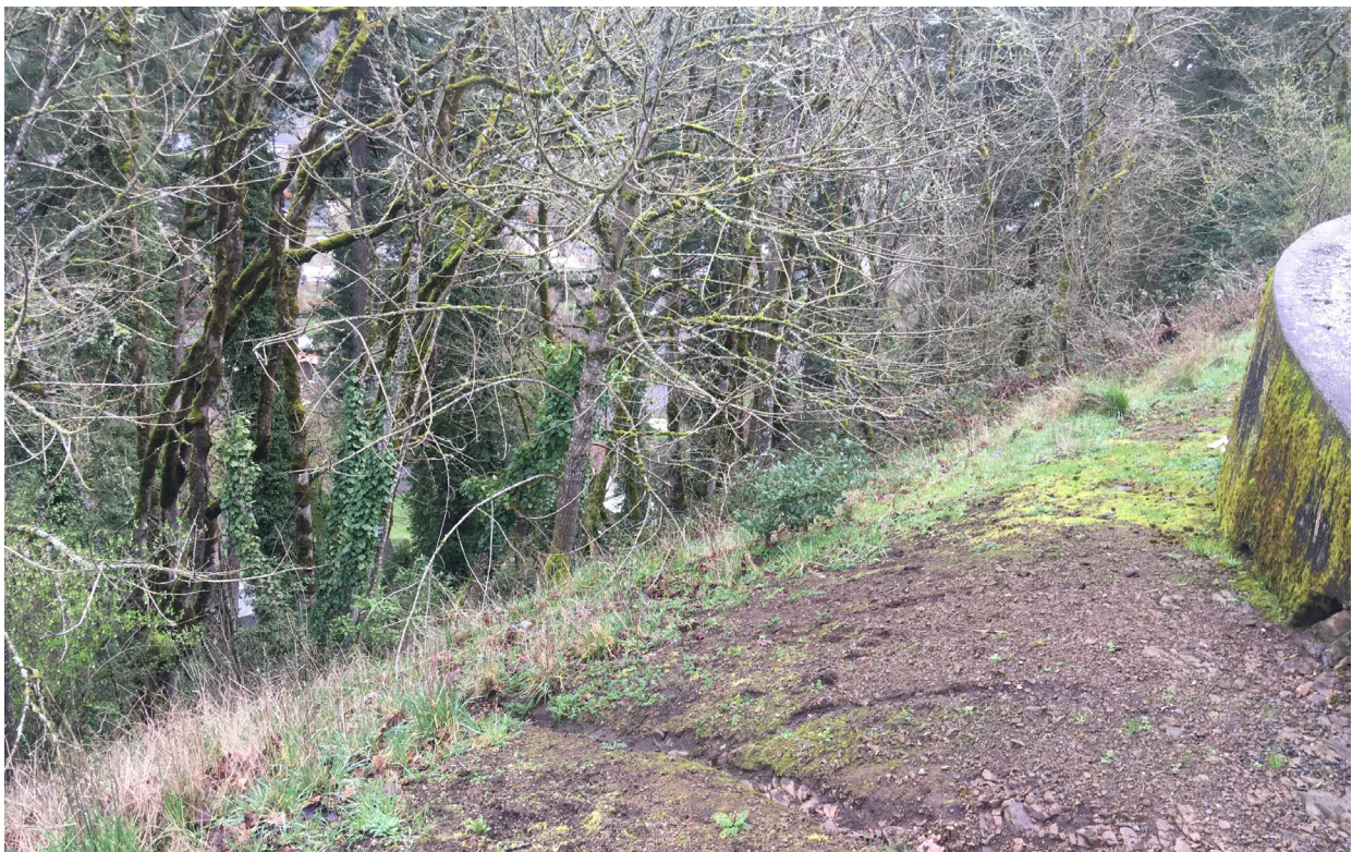
Kelly Butte Reservoir – Looking SE
