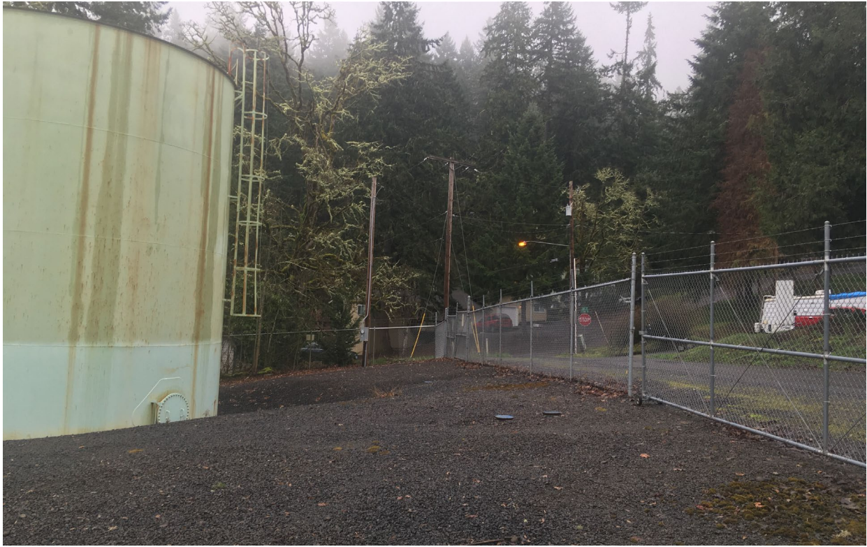
S 70 th Street Reservoir – Looking E
