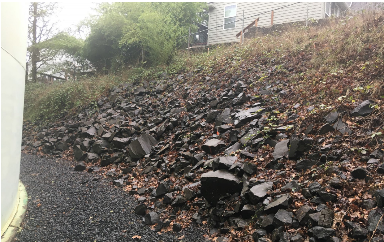
S 67 th Street Reservoir – Looking E
