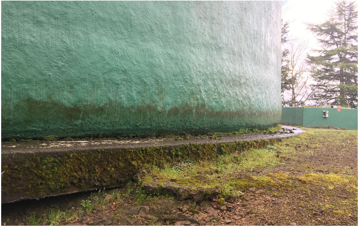
Kelly Butte Reservoir – Looking SE
