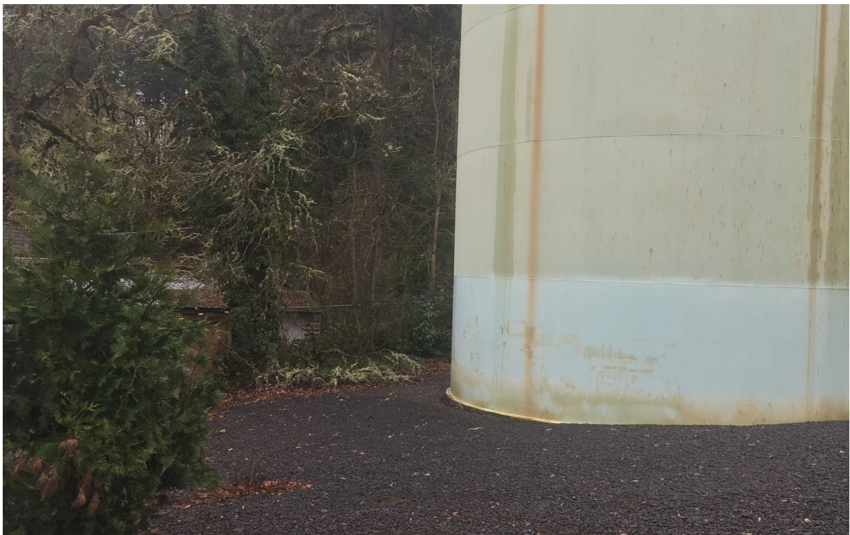
S 70 th Street Reservoir – Looking N
