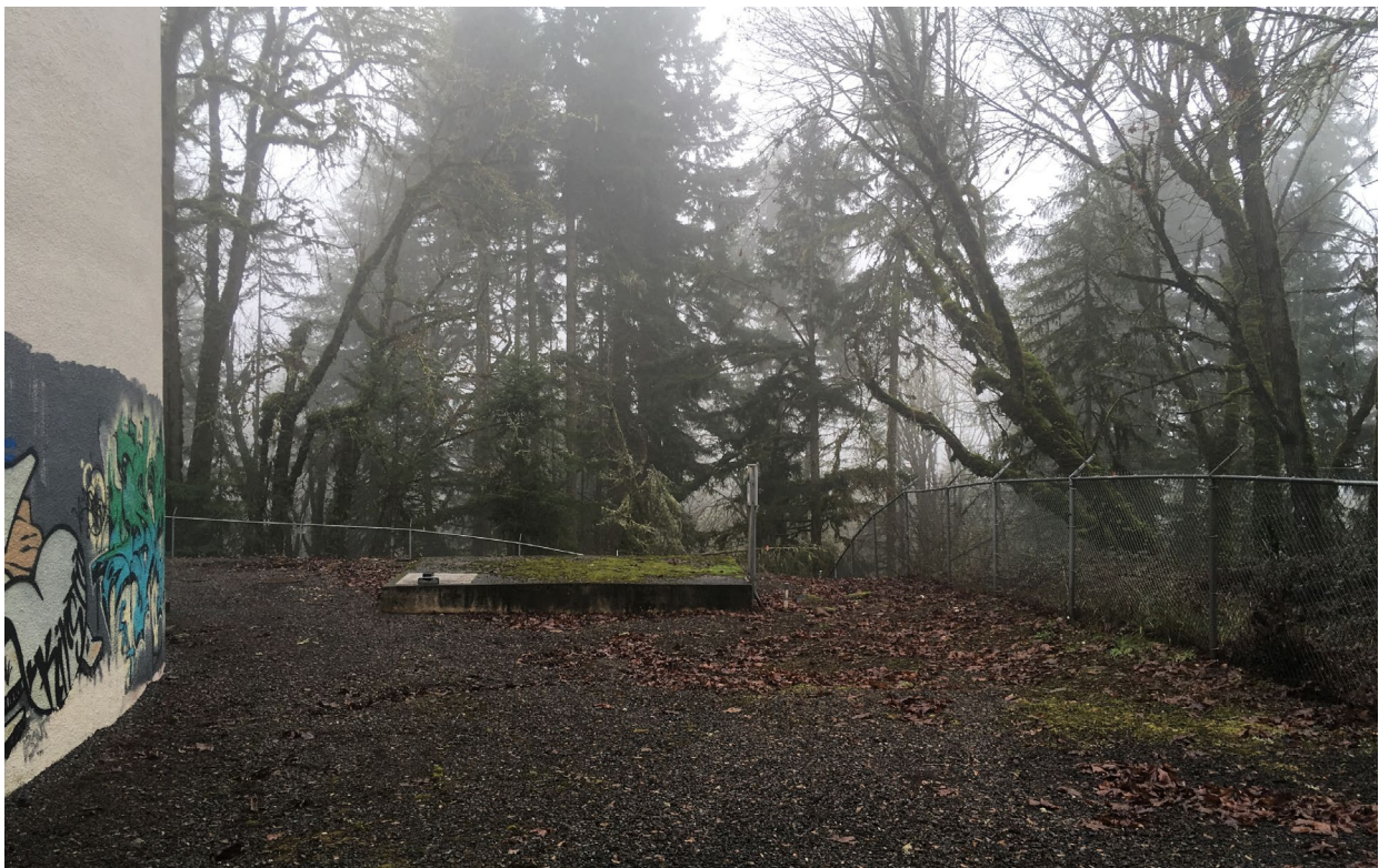
South Hills Reservoir – Looking NW
