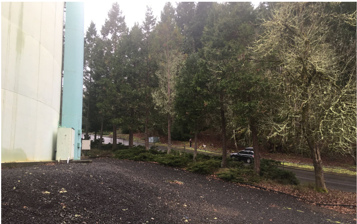
S 67 th Street Reservoir – Looking W
